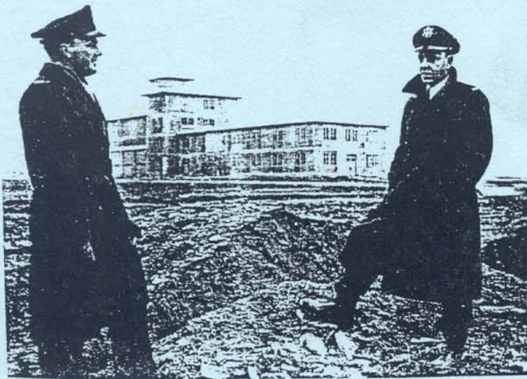
Approximately September, 1954. Still a lot of work to be done says Lt. Col. Charles J. Hoey, commanding the 7002nd Air Base Squadron on the new Chambley Base to Col. Robert R. Rowland, 21st Fighter Bomber Wing Commander, on an inspection tour from George AFB, Calif. Base Tower is in the background.
